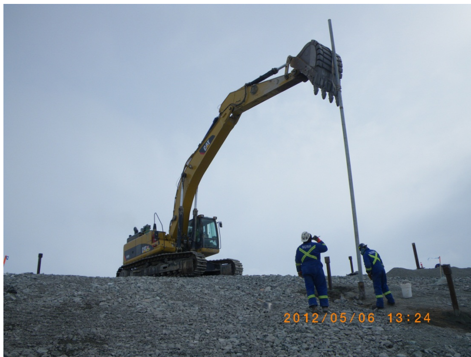
Photo 2: Installation of the last Deep Settlement Pipe into ND-DSP-070.
