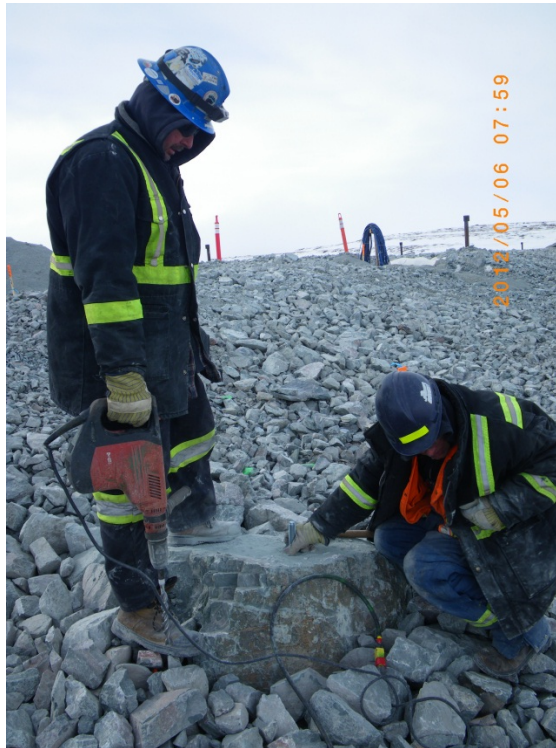
Photo 1: Installation of survey pins in the surface survey points.
